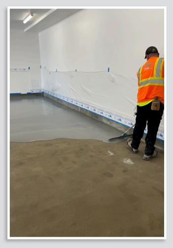
SPECLEVEL PCT-AGG is a cement-based, self-leveling polishable concrete topping designed for interior and exterior use.
